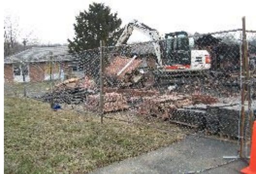
Taking down a wall - part 2
