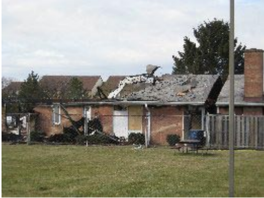
Removing the remaining roof
