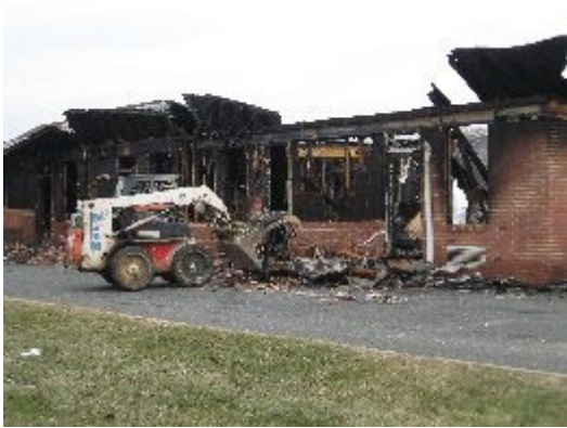
Removing debris outside rear wall
