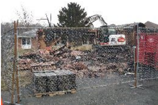
Taking down a wall - part 1
