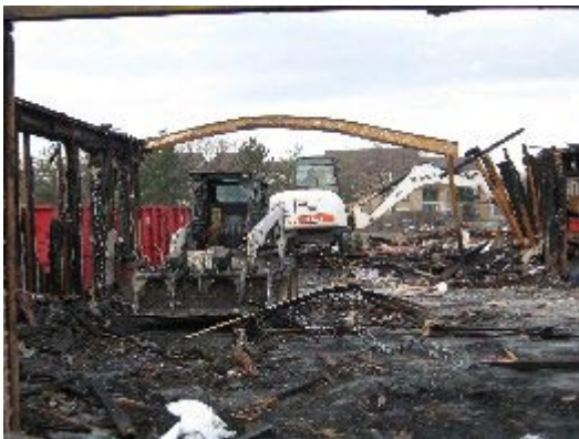
Steel I beam warped from fire
