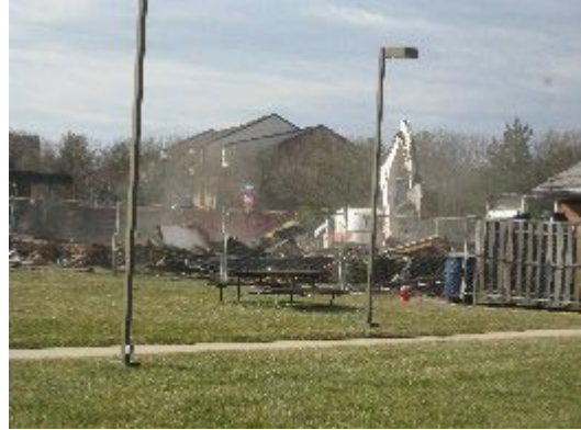
Taking down the last wall
